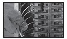
When moving two circuits with a shared neutral, they should be connected to adjacent positions (one above the other) in the transfer switch. That will assure that the two hot wires are on separate phases and will maintain their relationship to neutral.
